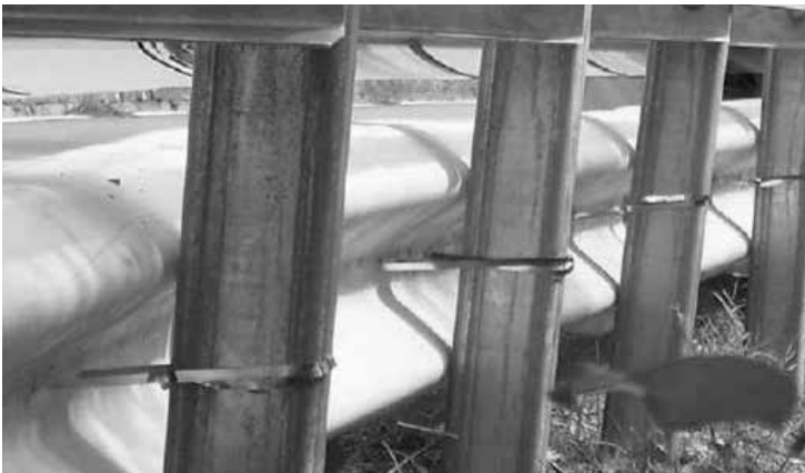
Figure 6: Pass cable ties through DR46 modules and attach to guardrail posts.
