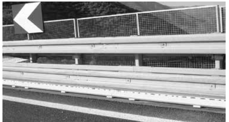
Figure 5: Approved custom installation using spacers
