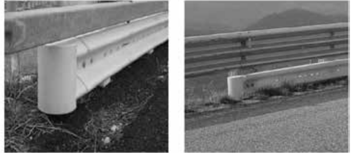
Figure 8: Connect DR46 MBA end modules
