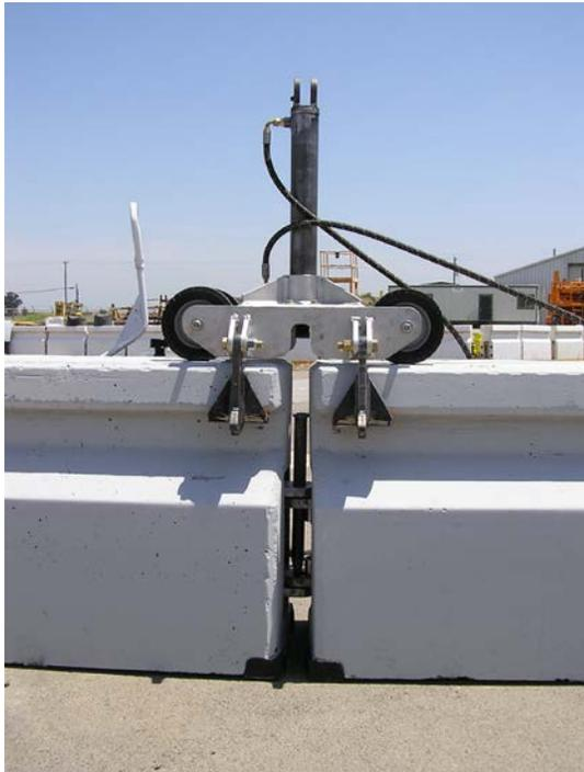
Hydraulic pin pusher mounted on the Barrier wall. It can be rolled to the next barrier connection after a new barrier set is put in place.
