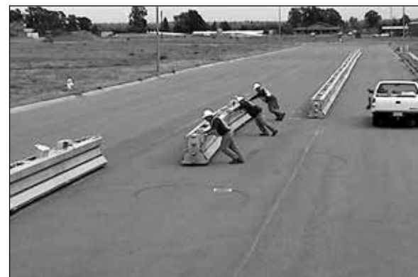
Figure 10. Relocate the section, or in this case Multi-section (56') to the desired position. Typically two people can easily control and move a single link section (28') and 3 people are typically used to move a multi-section (56') as shown above.
