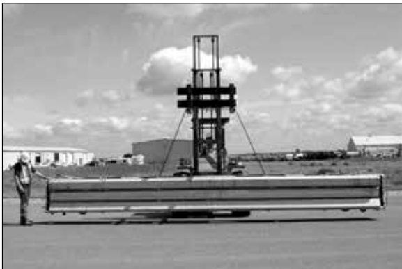
Figure 2. Use a crane, tractor or forklift to move the sections from the transport vehicle or trailer onto the job site
