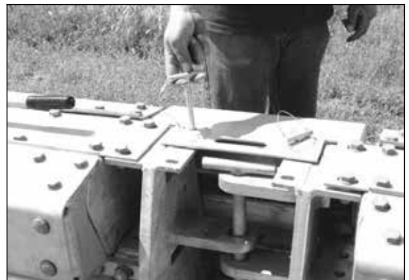
Figure 16: Rotate the cover up to the closed position and install the two keeper pins through the top as shown below.
