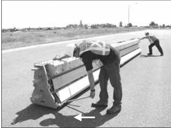
Figure 11. (QUICK TIP) If a section is difficult to get started moving, use the Hinge Pin as a lever to start the section moving.
