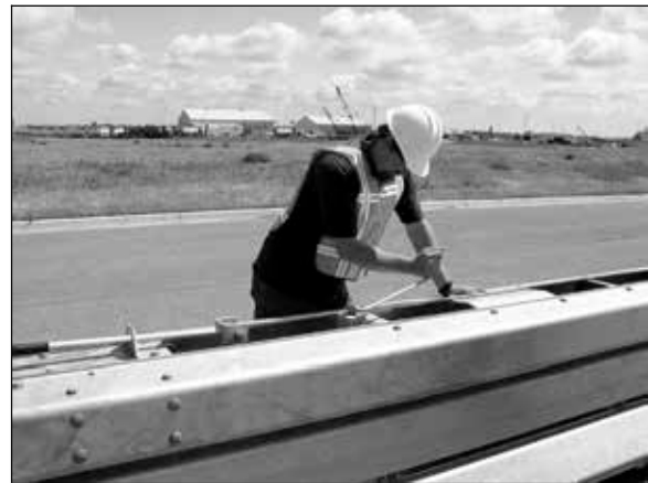
Figure 3. Manually jacking a section
