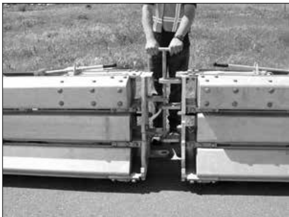
Figure 13. When all of the holes of the two section hinges are aligned, install the hinge pin. The pin must be fully installed.
