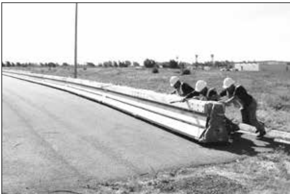
Figure 18. To deploy a barrier wall that is stored against a curb, move the end of the barrier out so that the truck can gain access.
