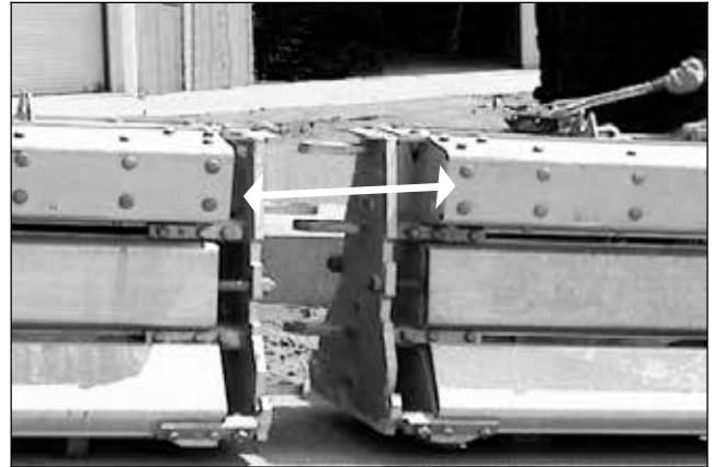
Figure 23. Use a winch or a “come along” as shown above to bring two sections together on a slope so that the hinge pin can be removed on installed.
