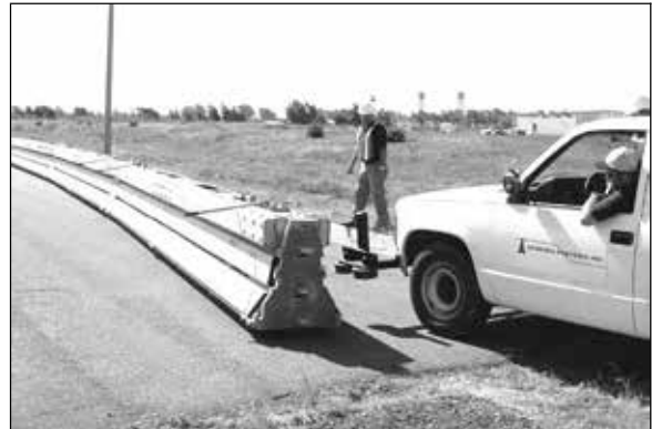
Figure 19. Push the barrier over with the vehicle as you drive along the side of the barrier. The tiller handles must be pointed in the direction of desired movement.
